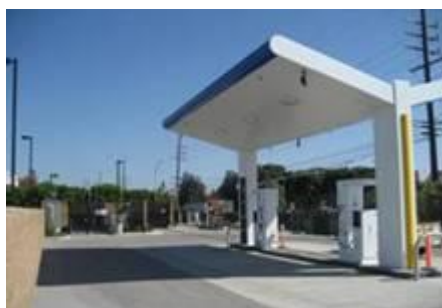
Figure 15: Torrance Pipeline Hydrogen Station
