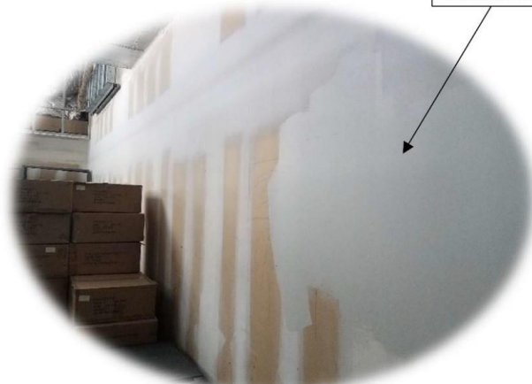
Figure 3: Photo of a partially painted wall system with paint (right side) covering joint compound and concealing where it was applied to the wall system
