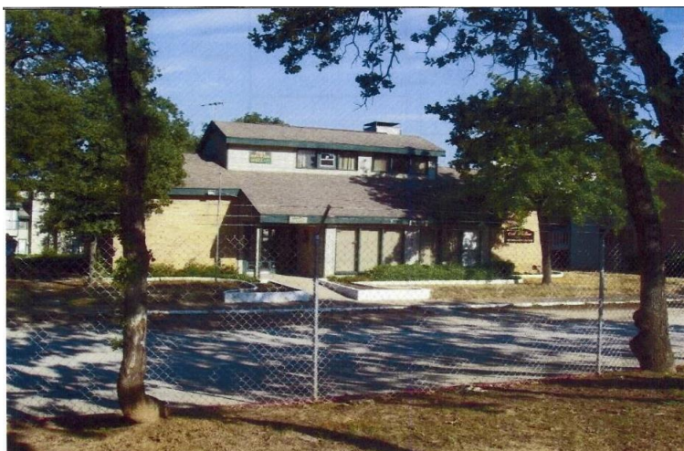
The AACM3 building with the asbestos-containing popcorn ceilings prior to demolition. (EPA photo)
