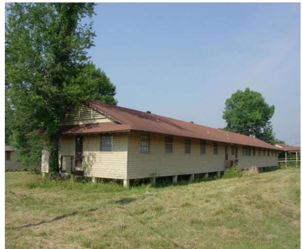
AACM1 building prior to demolition. (EPA photo)
