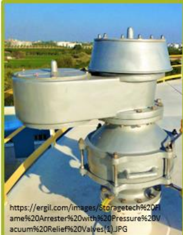
PRESSURE-VACUUM VENT Safety device that maintains pressure inside of tank
