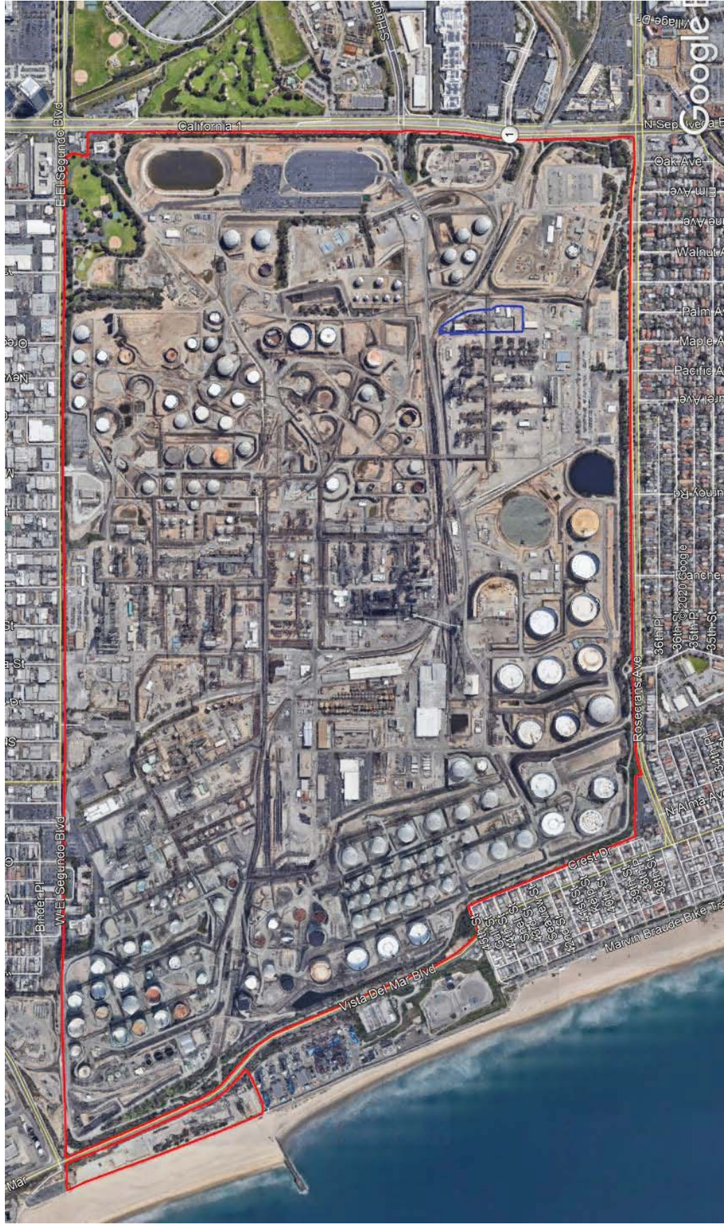
Figure 2-2 Air Liquide Facility Within the Refinery
