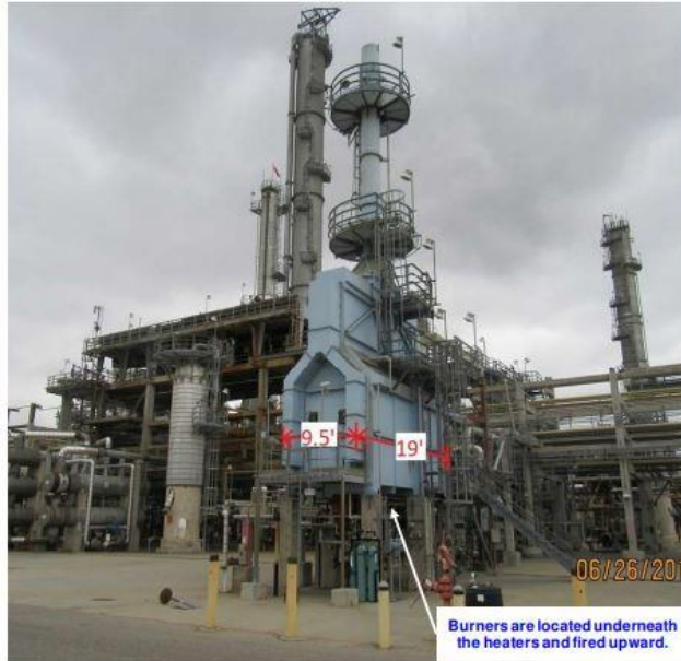
Figure 1-5 Upward fired natural draft cabin heater.
