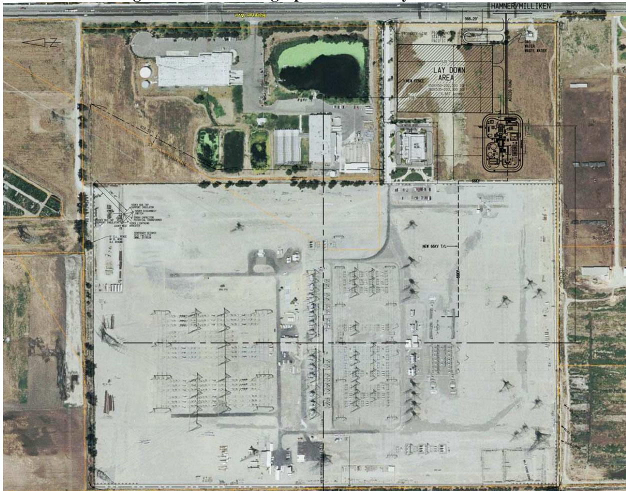
Figure 2 Aerial Photograph of the Facility with Plot Plan
