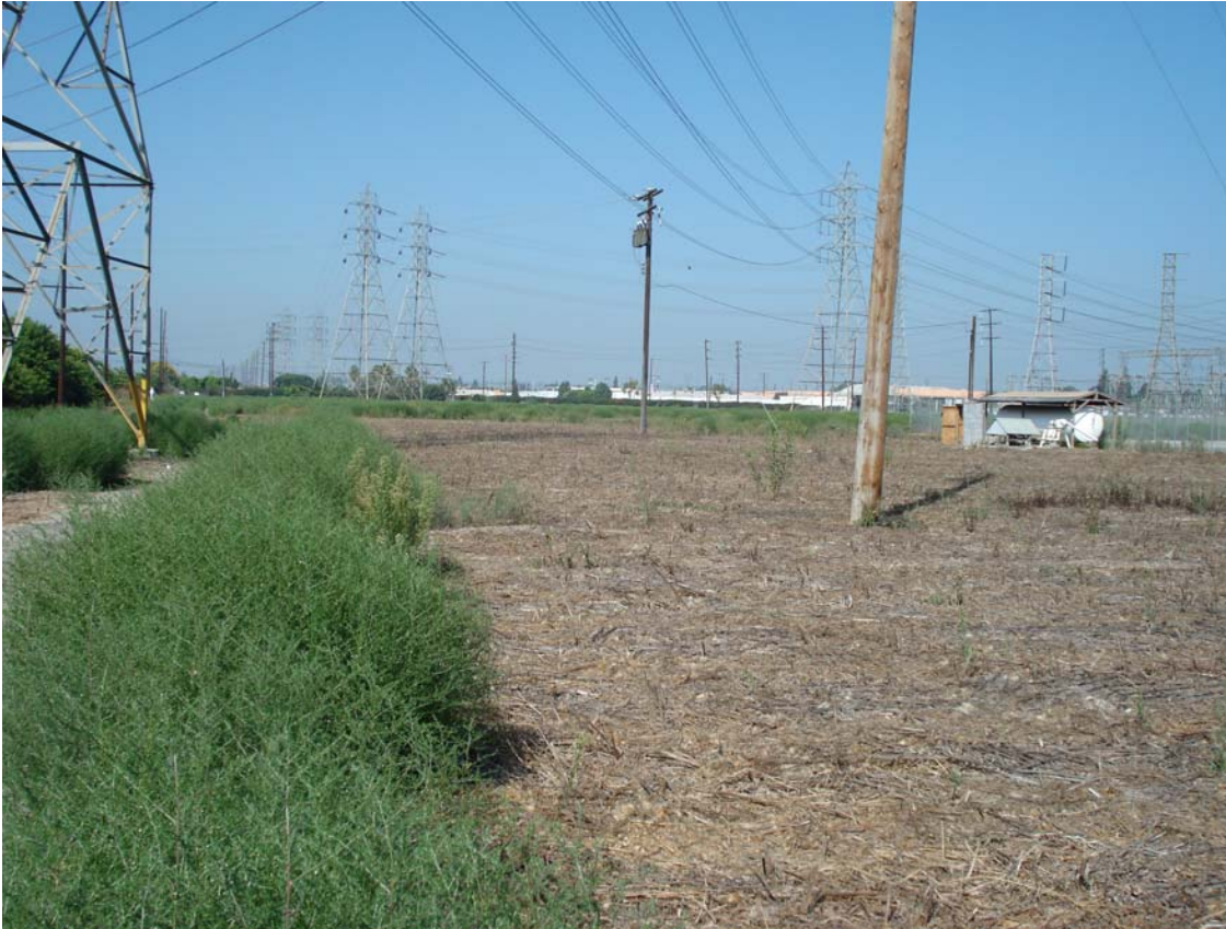
Figure 8: Looking northwest from the southeast corner of substation property.
