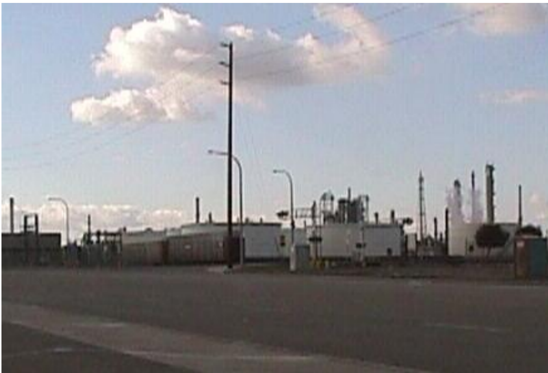
Figure 3-4.6: View of Refinery from south-eastern property line looking north-west.
