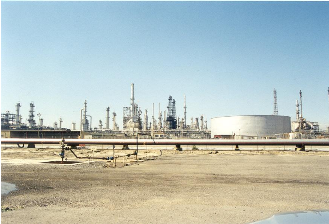
Figure 3-4.5: View of Refinery from the southern property line looking north.
