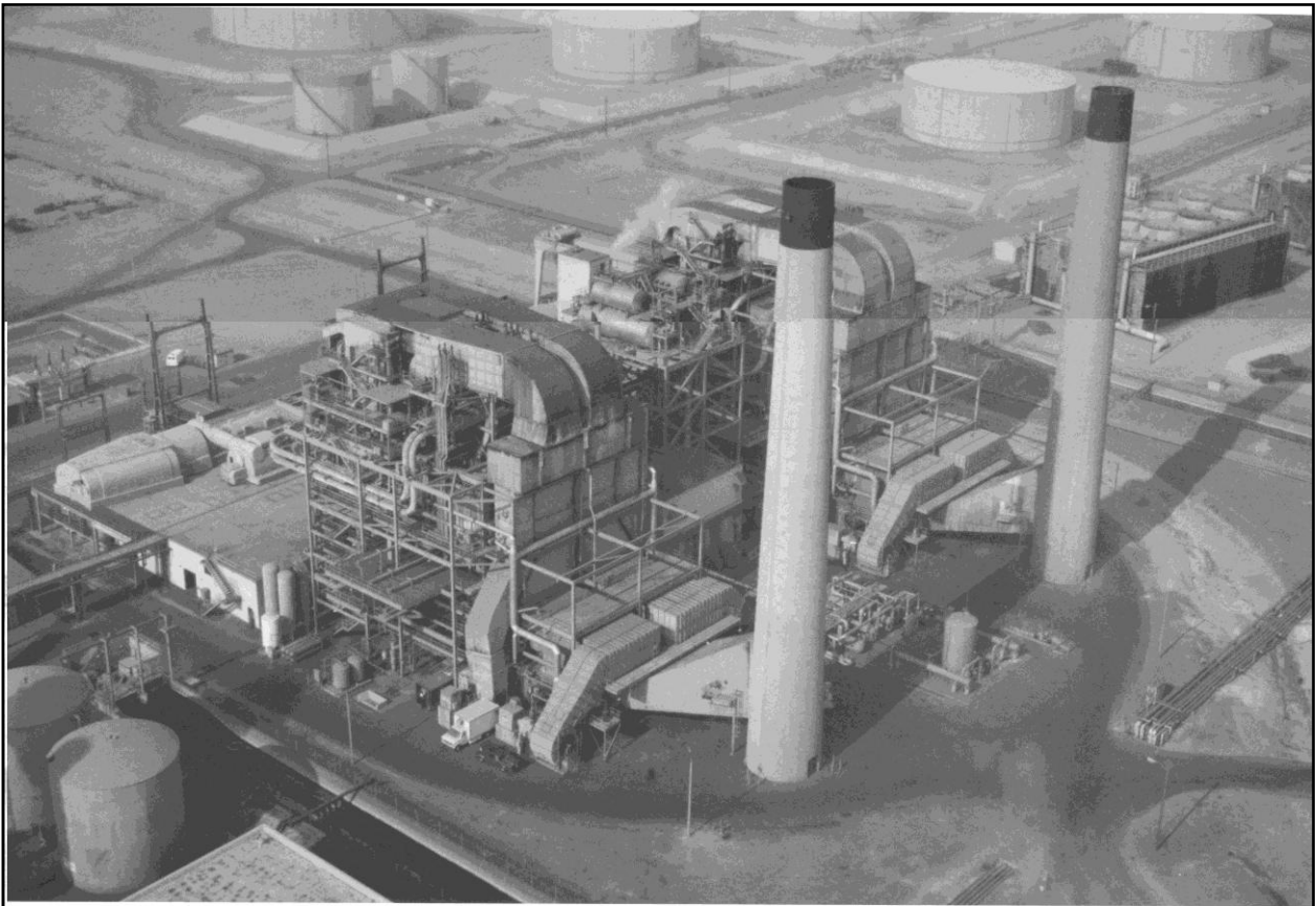
Aerial View of Units 3 & 4 of Etiwanda Generating Station
