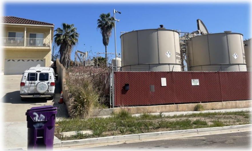
Street View of the Oil Site 3 and closest adjacent residence
