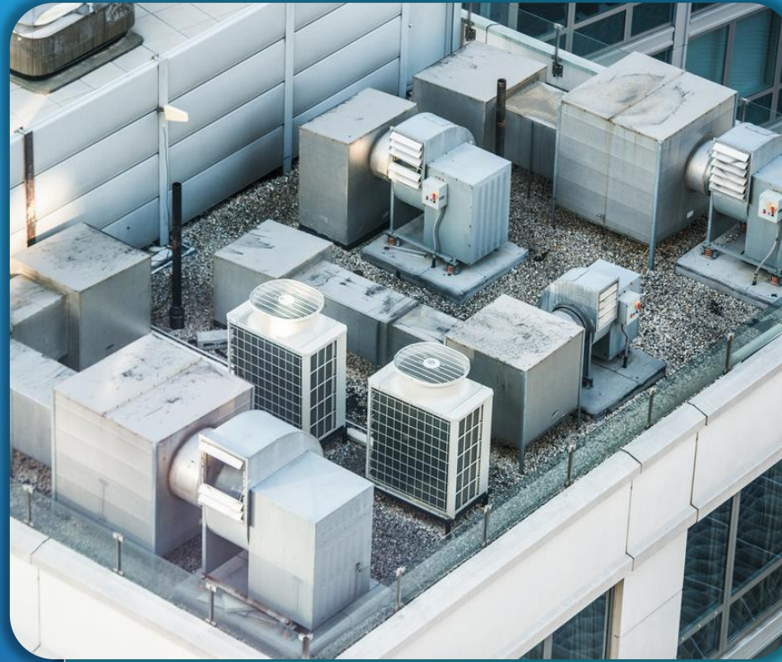
Commercial Combustion Water/Space/Heating/ Cooking/Others
