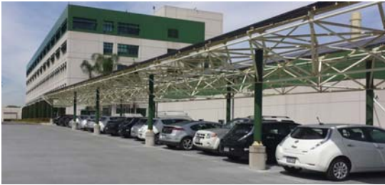
EV charging stations under the solar carport
