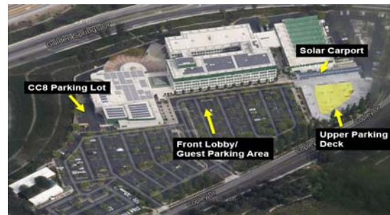
Locations of EV charging stations installed at South Coast AQMD headquarters
