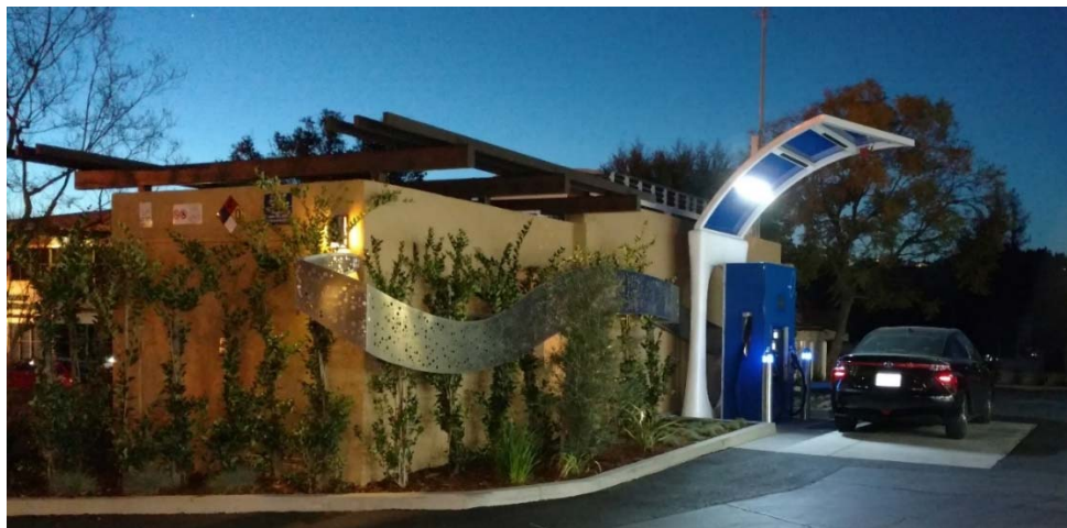
Figure 13: La Canada Flintridge Retail Hydrogen Station, Located at Arco Gas Station
