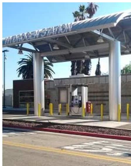
Figure 2: Hydrogen Produced with Hydrogenics Electrolysis System at CSULA
