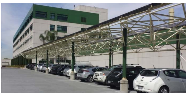
Figure 11: Existing Level 2 Chargers under SCAQMD's Solar Carport
