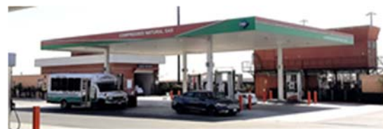
Figure 2: CNG Station after expansion
