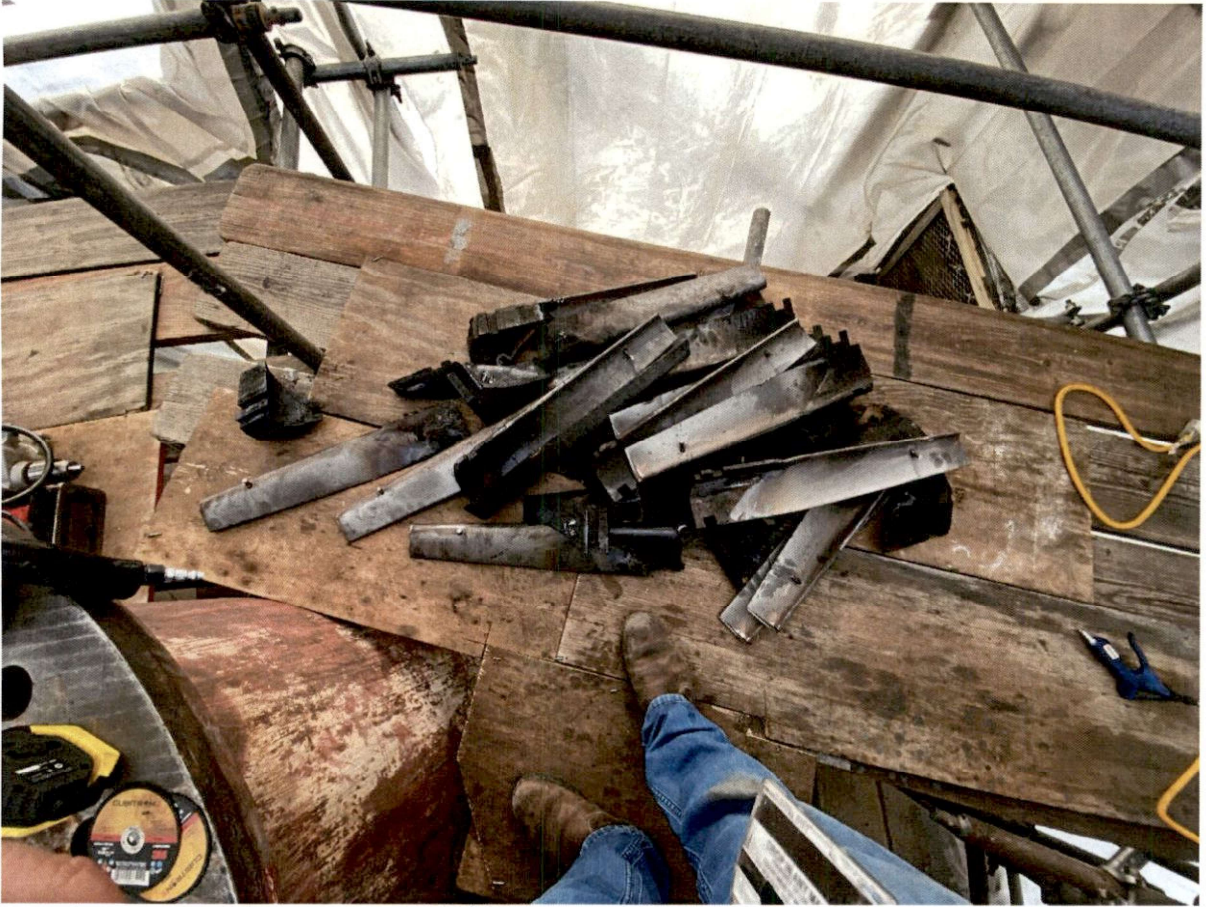
May 9 th , 2023 – Removed Damaged Top Case Stationary Blades, Stage 5
