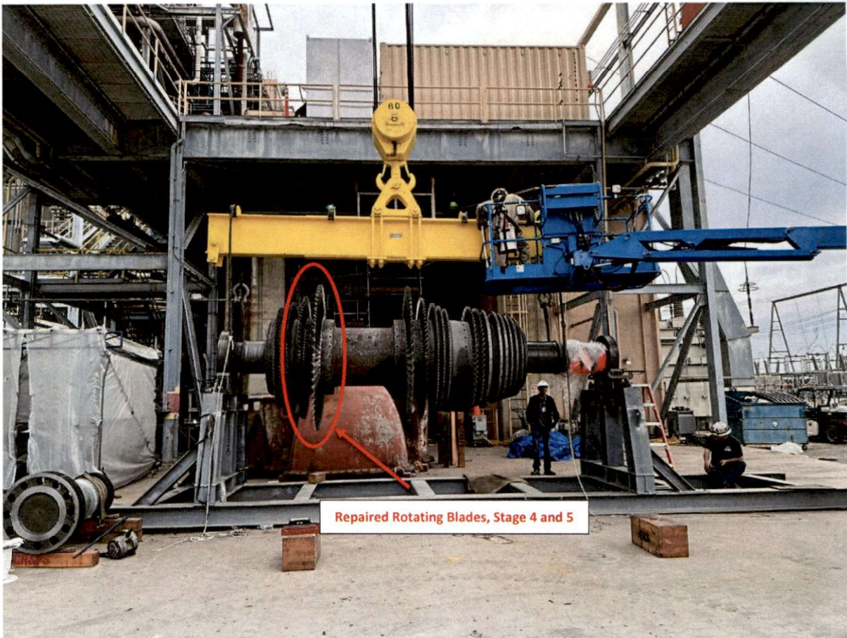
July 23 rd , 2023 - Repaired Rotor on Stand
