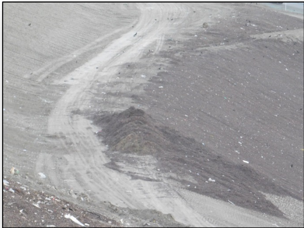
Wood Waste Applied for Erosion Control
