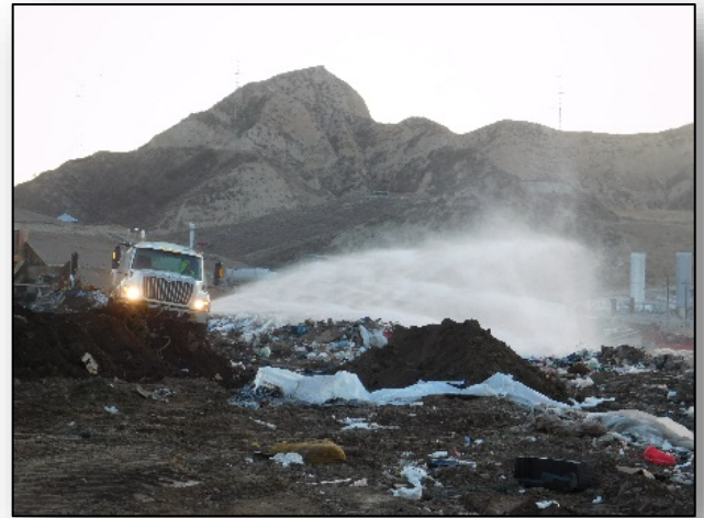
Water Truck Applying Neutralizer
