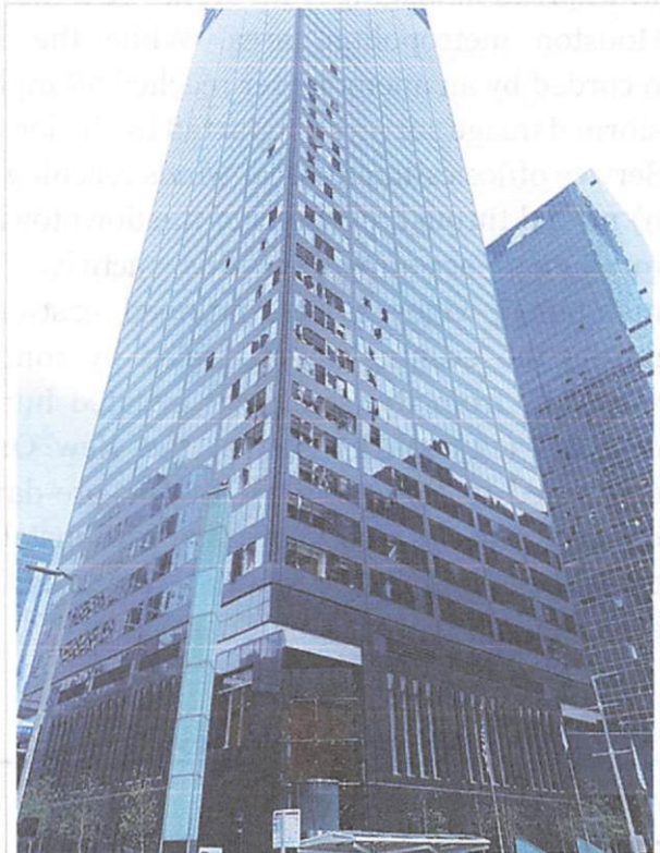
Windows blown out of CenterPoint Energy Plaza in Houston
