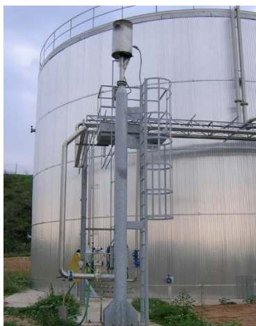
Figure 3-1. Non-Hydrogen Clean Service Flare (LPG Flare)
