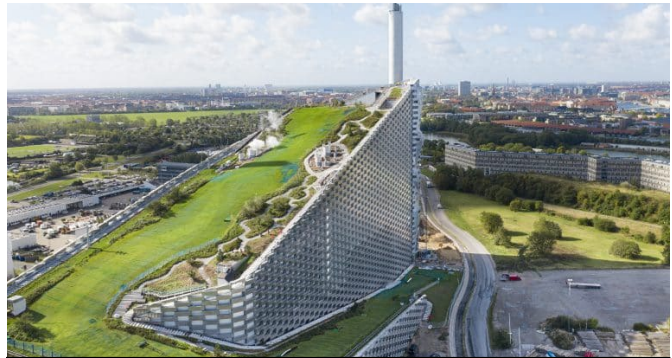
Figure 2-3: Amager Bakke Waste-to-Energy Plant. https://a-r-c.dk/amager-bakke .
