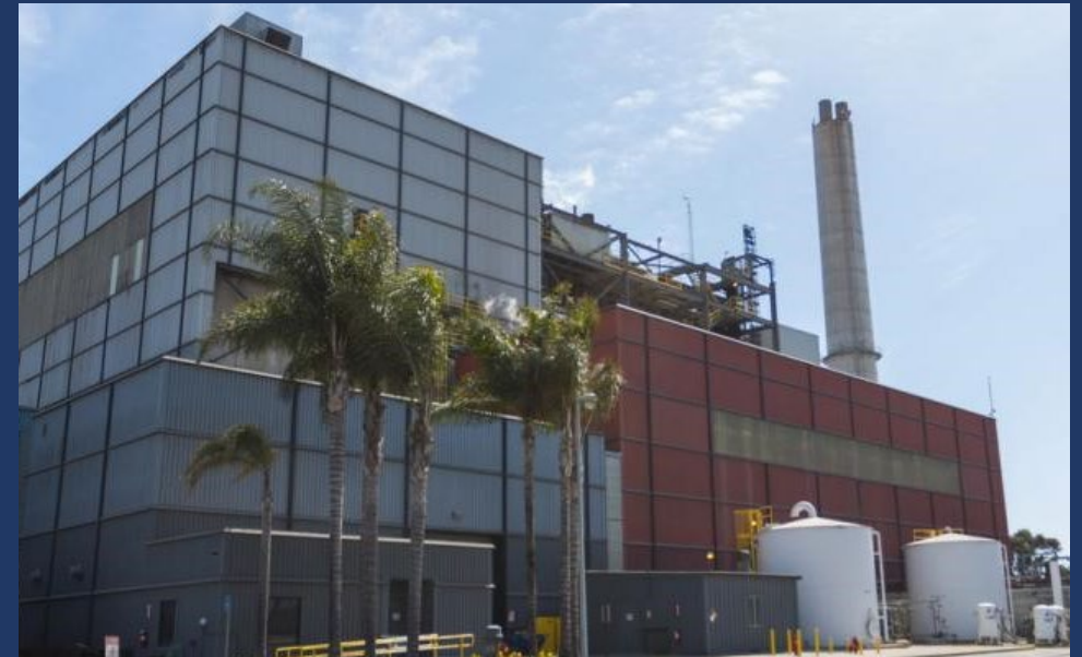
Image: SERRF facility in Long Beach
