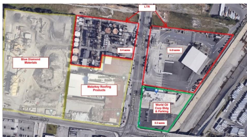
Figure 2-13: LTR dba World Oil Refining Facility
